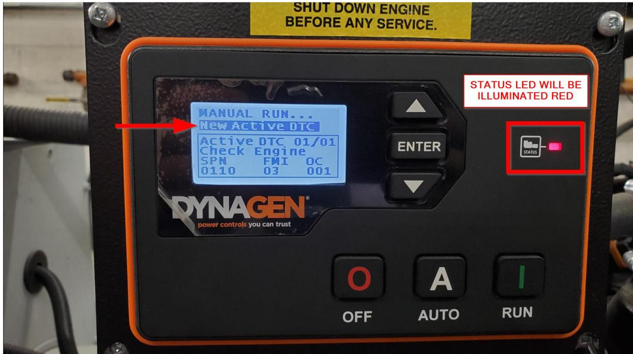
Figure 3. Example: DTC 110.03 fault is set while the engine is running normally
