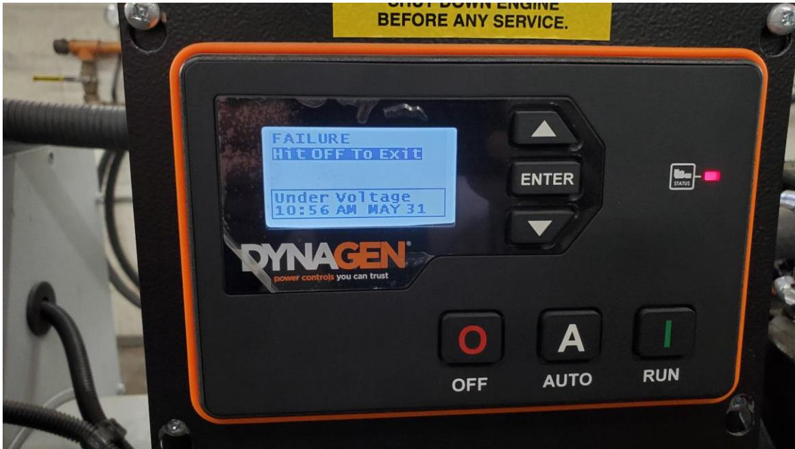
Figure 4. Front panel display after engine has shutdown by ECU shutdown
