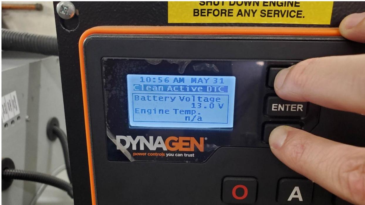
*Figure 2. Front panel display during Clear Active Faults action*
