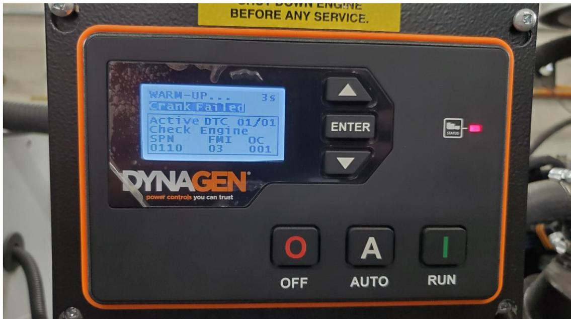
Figure 5. Engine restarted and shut down again by ECU; root cause of fault not corrected
